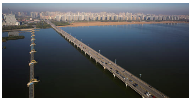
The lifting engineering of Yihe Bridge, Beijing Road, in Linyi, has a total length of 1210.72 meters, a lifting height of 3.1 meters, and a lifting area of 2680 square meters. The lifting engineering of Yihe Bridge in Shandong province is the lifting and reconstruction engineering of single bridge with the largest synchronous lifting area and longest length in China.
