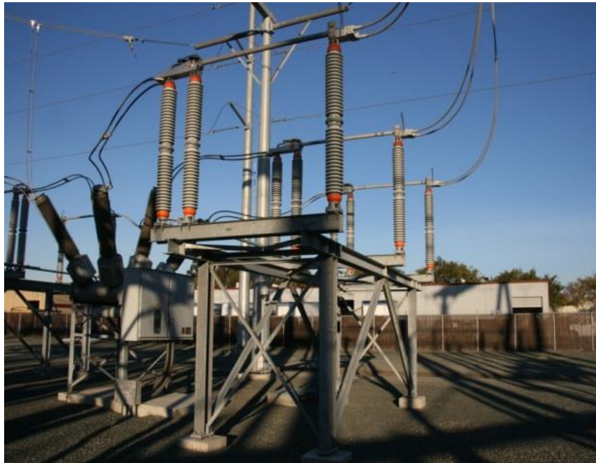
230 kV Disconnect Switches in Substations
