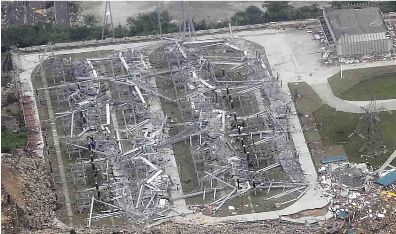
Ertai Shan Switchyard (220kV) Destruction ( PGA \sim 0.5g ), Yingxiu Town Wenchuan Earthquake, China, May 12, 2008 [Photo credit: Q. Xie, Tongji University]
